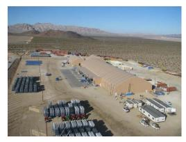
The heliostat assembly building with mirrors ready for transport to the solar fie
